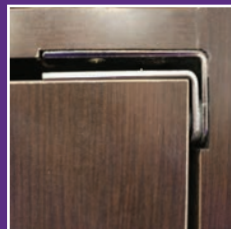
Heavy-duty swing door hinge
